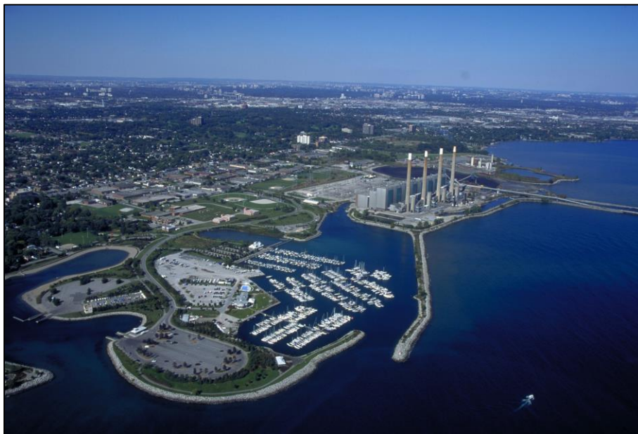
Figure 12: Lakeview Generating Station Site
